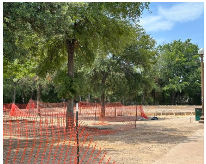
Work is underway at Daggett Park!
